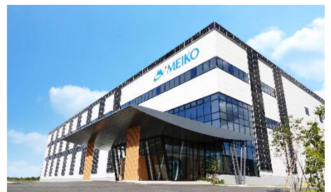
<Tendo Factory: 170kW Self-Consumption Solar Power Generation System>
