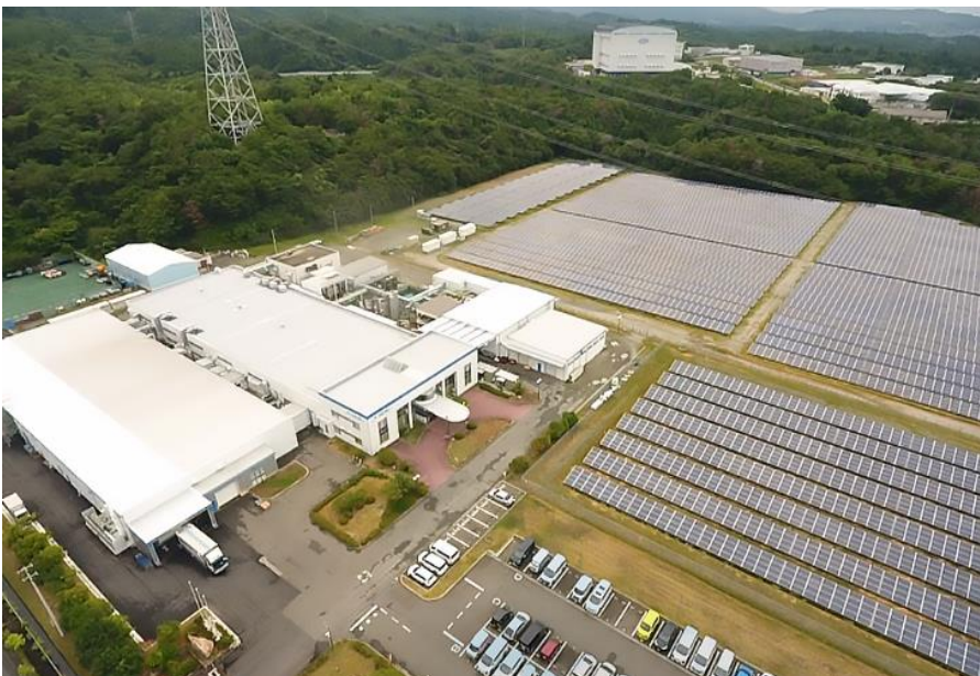
<Fukushima Factory: 532kW Self-Consumption Solar Power Generation System & Solar Park Fukushima>
