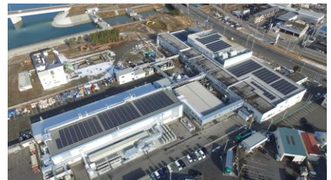
<Ishinomaki Factory: 383kW Self-Consumption Solar Power Generation System & Solar Park>
